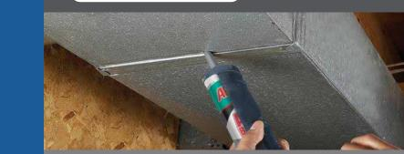
High quality universal hybrid sealant & adhesive based on MS polymer
