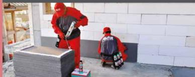
One component minimal expanding aerosol polyurethane adhesive foam curing swiftly with moisture. Providing very fast and powerful adhesion for various construction materials, especially highly recommended for heat in-
