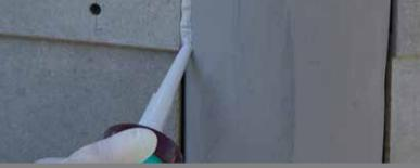
One-component, medium-modulus polyurethane sealant that cures on exposure to atmospheric humidity. It possesses excellent adhesion to all typical construction materials such as cement based materials, brick, ceramic,wood, galvanized and painted sheet iron and various plastics.
